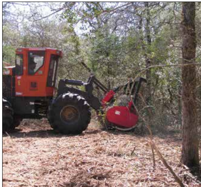
Figure 7. Mechanical brush treatments have the immediate effect of reduced canopy cover, but can cause significant soil disturbance and some species will vigorously resprout. A rotary mulcher is pictured here. (Photo courtesy Tim Siegmund, Texas Parks and Wildlife)
